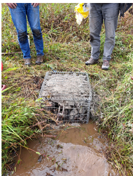
A gabion will provide a strongpoint to moor the boat at Loch Nell
